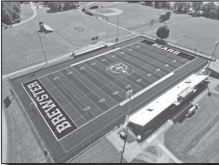
The new turf field on the Brewster Schools campus is complete. With the ground leveled, a sub-base installed, turf laid, lines painted and the Brewster Bear logo placed at mid-field, it is ready for fall games.
